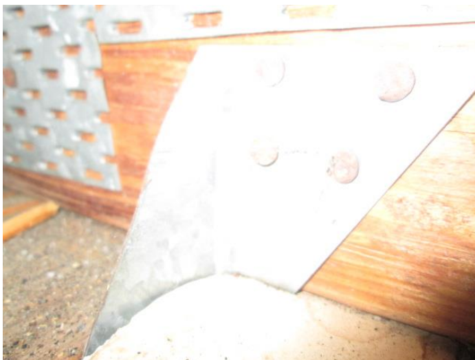
Roof to Wall Attachment
