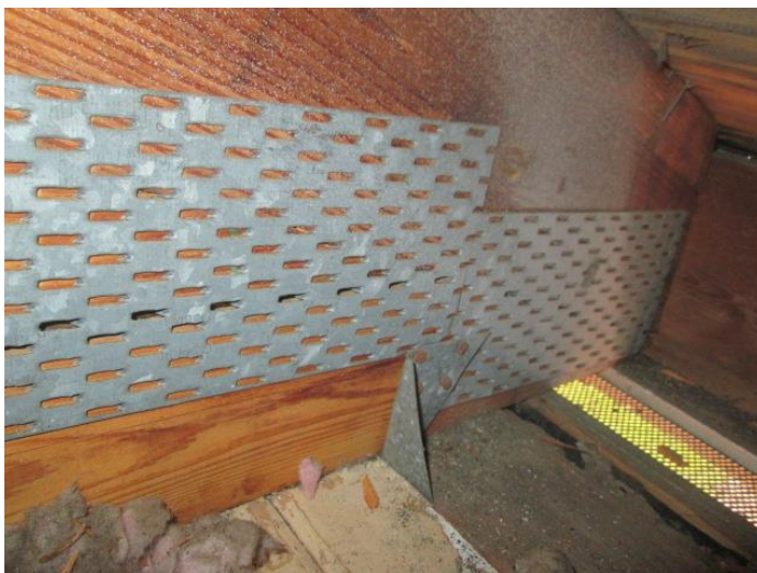
Roof to Wall Attachment
