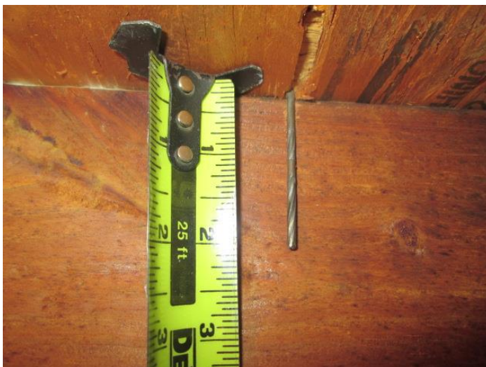
Roof Deck Attachment
