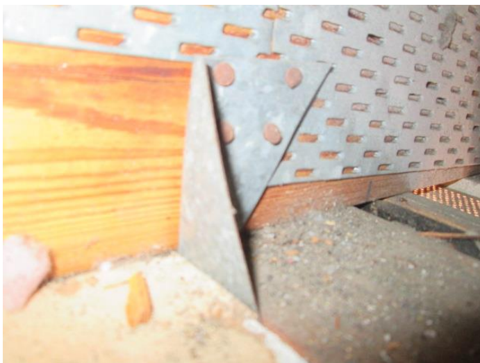
Roof to Wall Attachment
