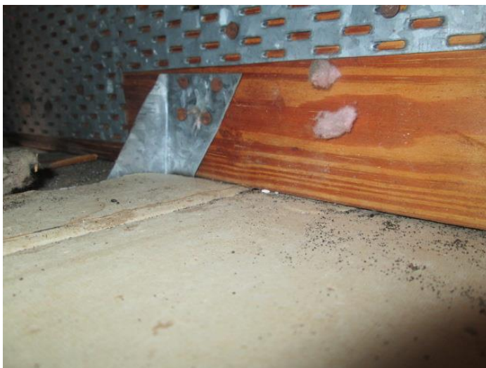
Roof to Wall Attachment
