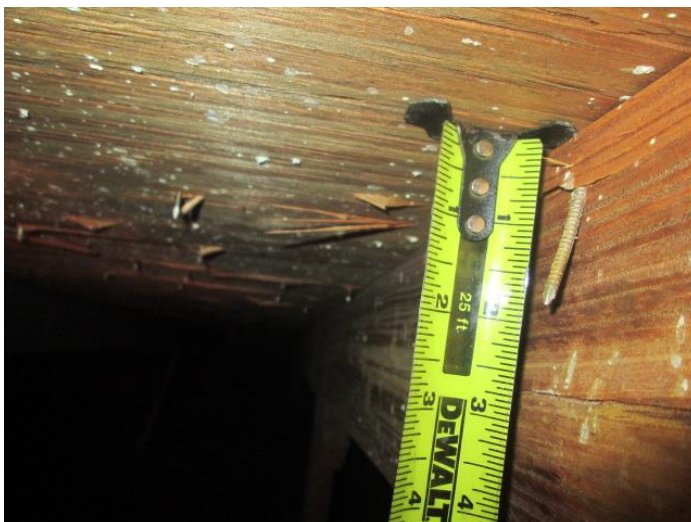
Roof Deck Attachment
