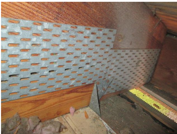
Roof to Wall Attachment
