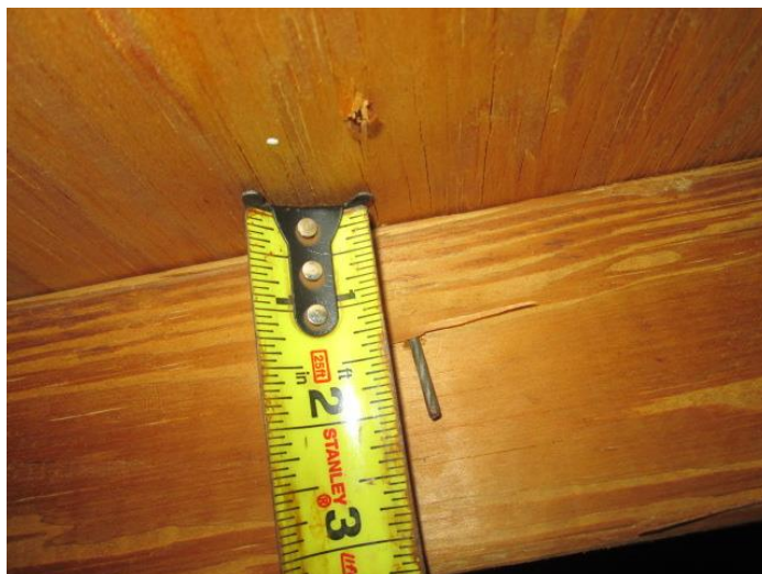
Roof Deck Attachment
