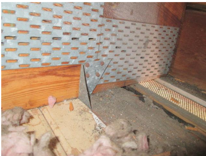
Roof to Wall Attachment
