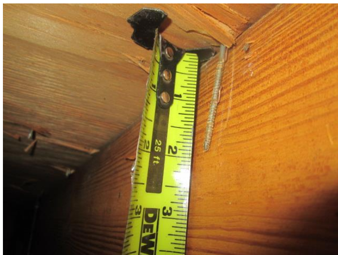
Roof Deck Attachment
