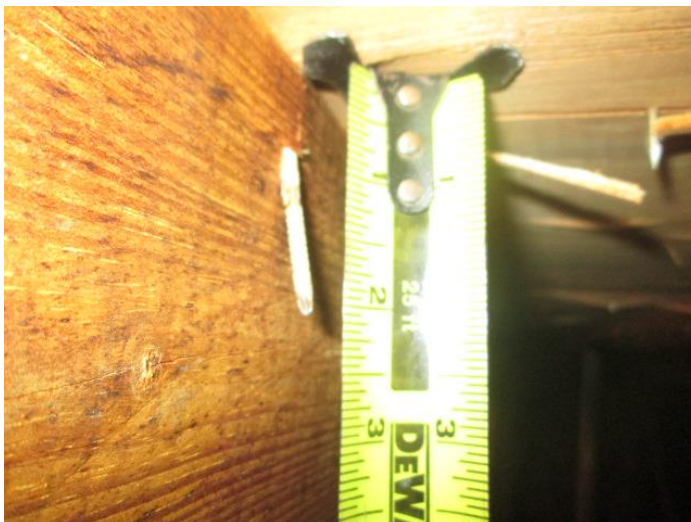
Roof Deck Attachment
