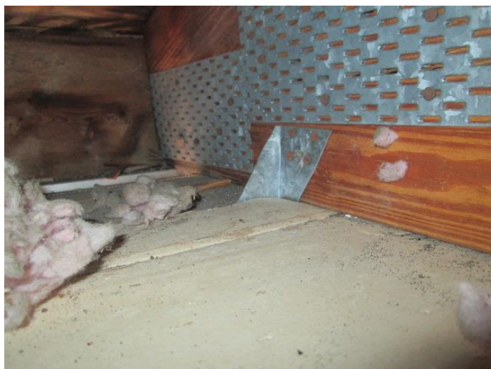
Roof to Wall Attachment
