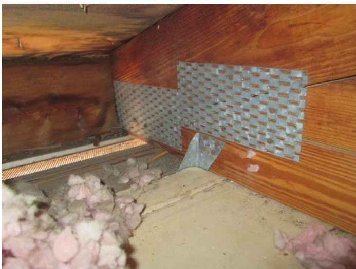
Roof to Wall Attachment
