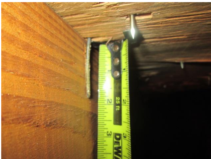
Roof Deck Attachment
