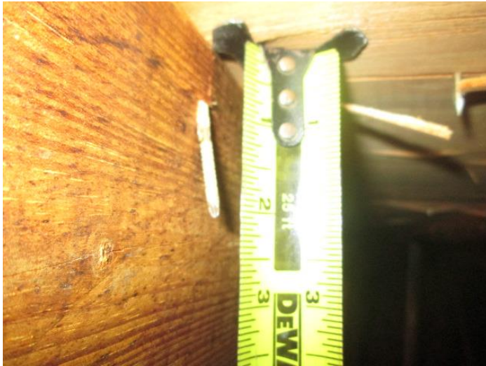
Roof Deck Attachment
