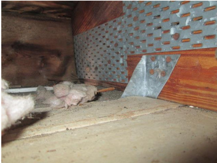
Roof to Wall Attachment
