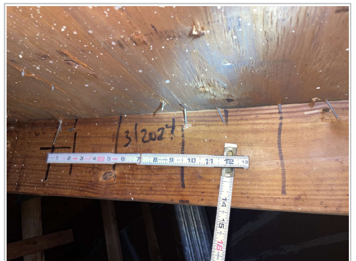
8d Nails within 6"
