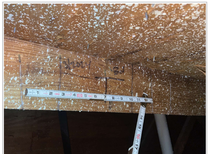
8d Nails within 6"
