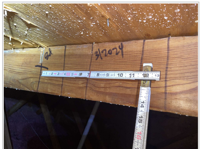
8d Nails within 6"
