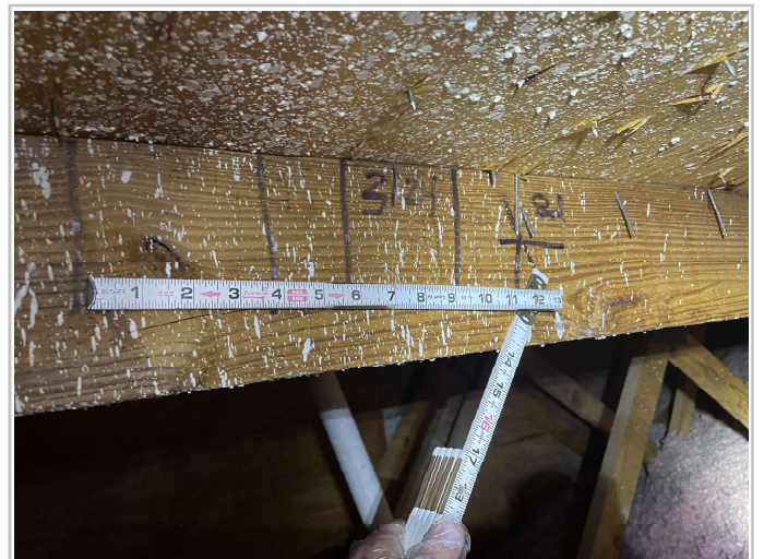
8d Nails within 6"
