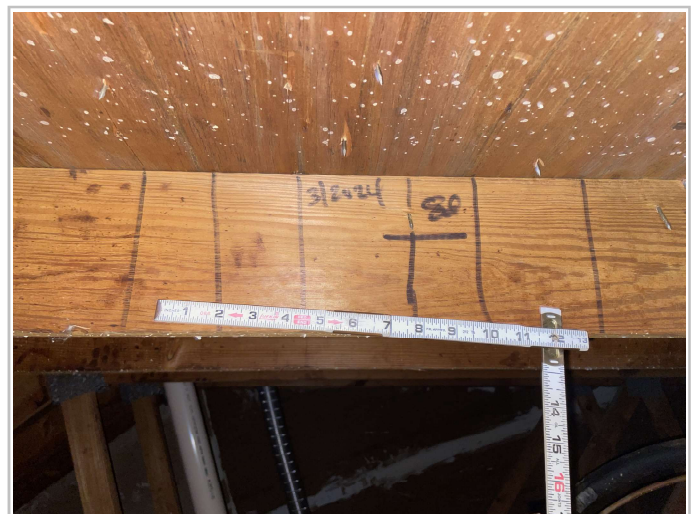
8d Nails within 6"
