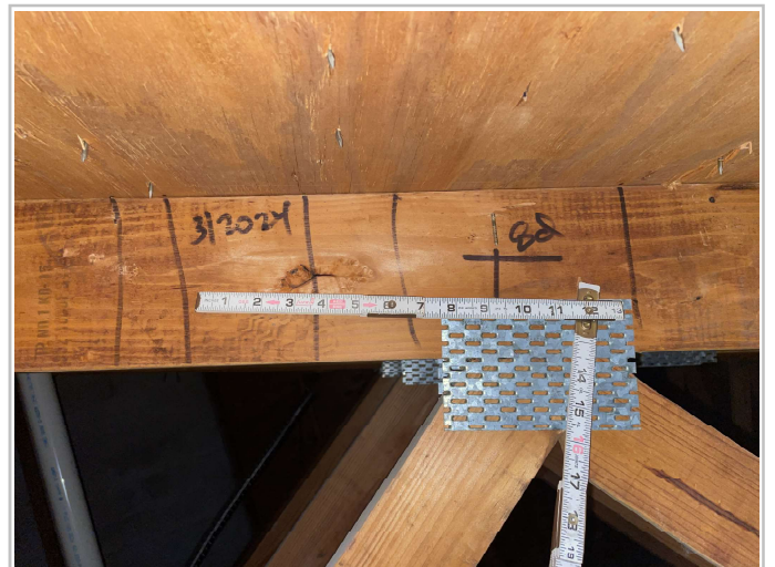
8d Nails within 6"
